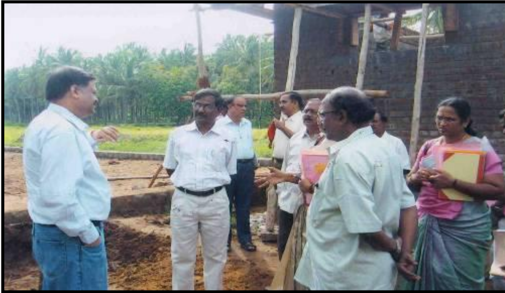
Agri Business Centre under construction at Thimanguthu, Pollachi and World Bank Agri Marketing Consultant in conversation with farmers and officials at site.
